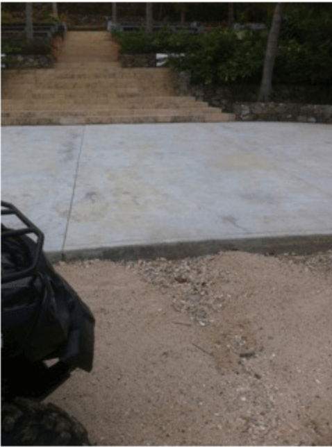
step in front of nursery; Ion should paint the floor with fish stencil design
