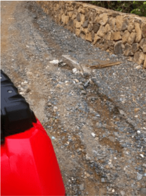
drainage for roads
