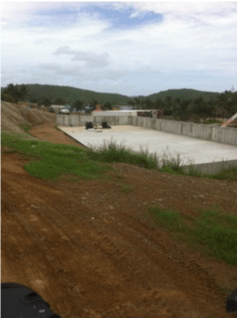
tennis fencing and paint and plaster of walls
