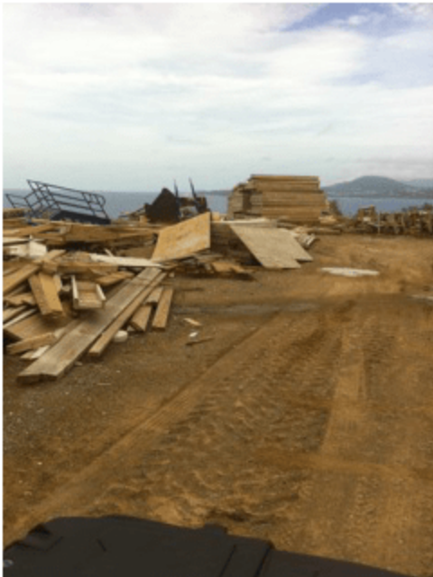
Clean up top of hill
