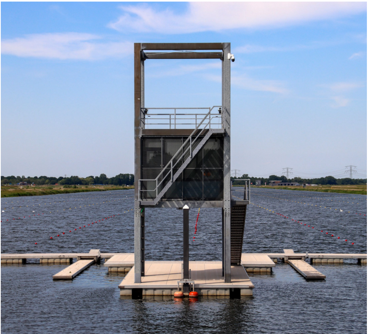
↑ A rowing facility in the Eendragtspolder water storage facility for flood prevention: Rotterdam, the Netherlands
